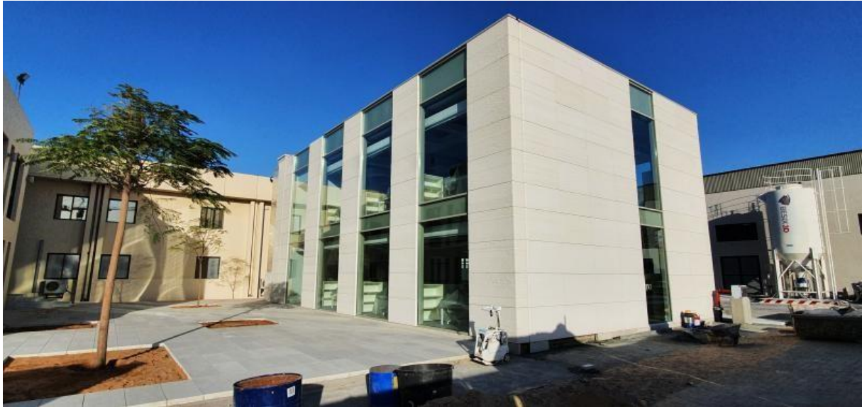
HQ Besix Dubai, partially 3D printed
