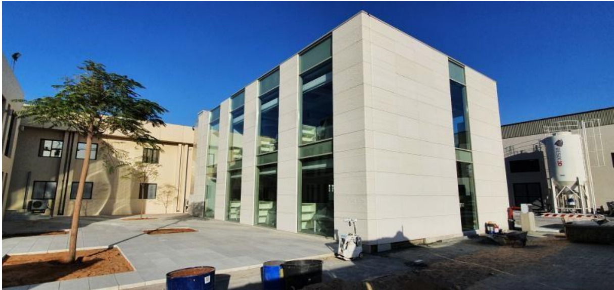
HQ Besix Dubai, partly 3D printed
